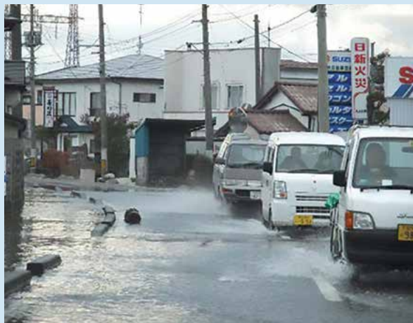
Photos 3.6: Inundation of Coastal Areas due to Subsidence Caused by the 2011 Great East Japan Earthquake (Ishinomaki City). A coastal road was submerged by seawater even in the normal high tide. (Cited from MLIT (2012))
