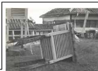
Fallen meteorological screen in Kamezaki weather observatory
