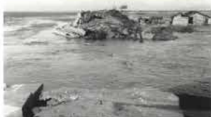
Breach of bank: Tenposhinden
