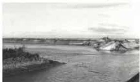
Breach of bank: Kawakitashinden
