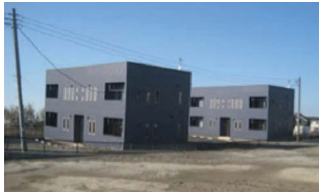
Figure 2.9 Subsidence of houses from liquefaction
