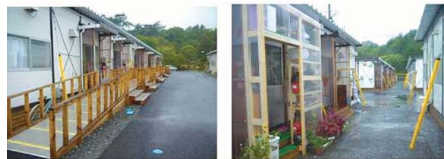
Temporary houses in Ofunato, Iwate; and Onagawa, Miyagi
