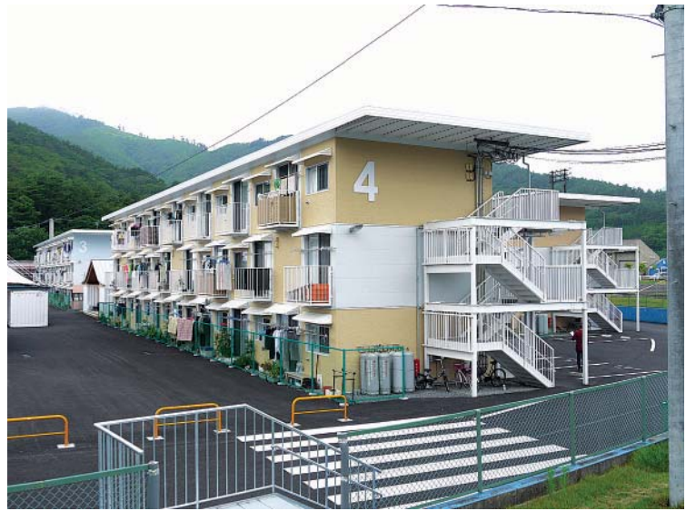
Figure 22.6 Multiple-story temporary housing made with stacked containers
