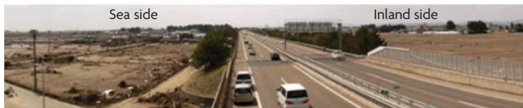
Figure 4.1 East Sendai Expressway
