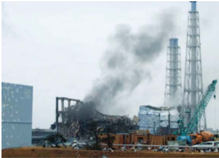
Figure 5.9 Fukushima Daiichi Nuclear Power Station
