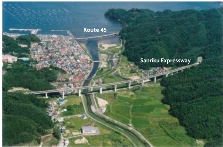
Figure 4.2 The Sanriku Expressway was built with tsunamis in mind
