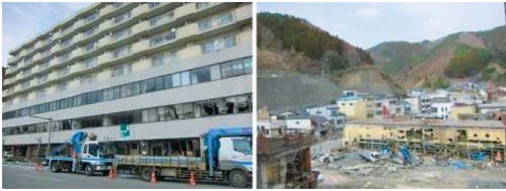
Figure 27.4 Designated evacuation building (left) and evacuation road (right) in Kamaishi
