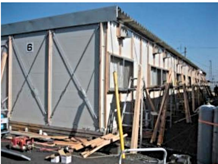
Figure 22.5 Improvements to temporary housing—adding insulation to the walls and double-pane windows
