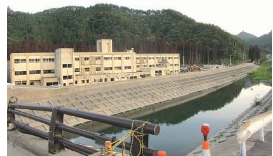
Figure 8.2 Kamaishi-higashi Junior High School (top) and Unosumai Elementary School (bottom) are located near the sea
