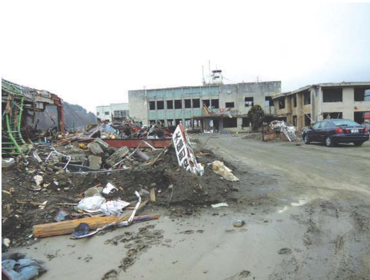
Figure 17.1 The municipal office in Otsuchi Town was damaged by the tsunami
