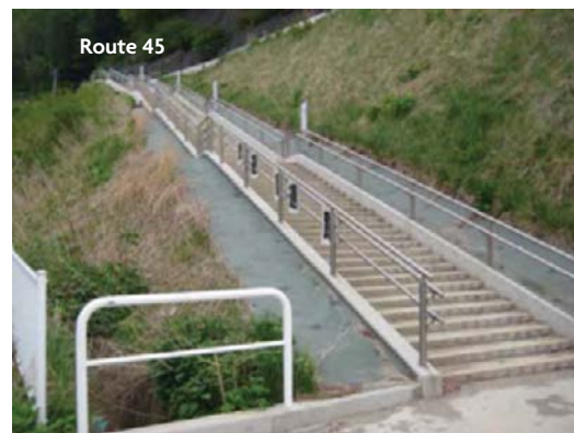
Figure 4.4 Evacuation stairway at the Omoto Elementary School
