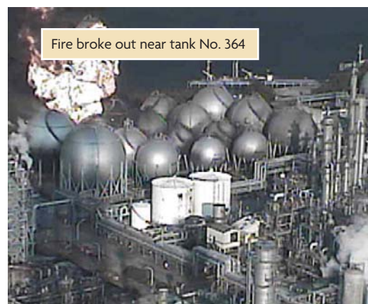
Figure 5.5 Leaked LPG catches fire at a refinery
