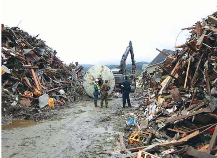
Figure 20.5 Clearing of roads
