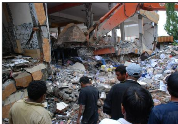
Figure 3: Debris removal after the earthquake
