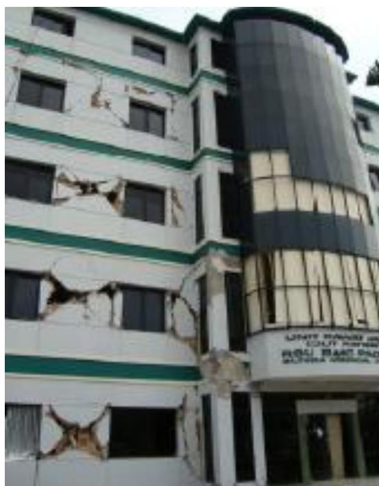
Figure 4: Earthquake resistant building construction is required to reduce future damages
