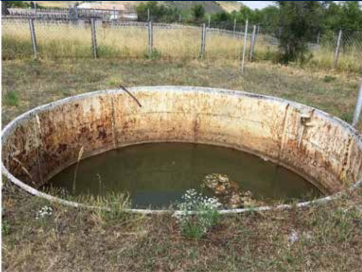
PHOTO 6. EVAPORATION TANK AT AN OBSERVING STATION, LAKE SEVAN STATION
