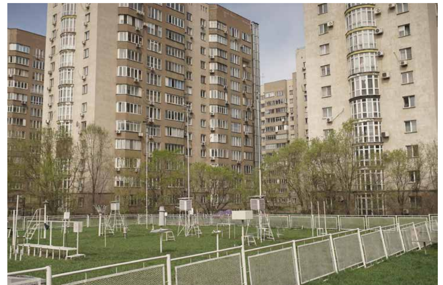
Development near the Almaty meteorological station
