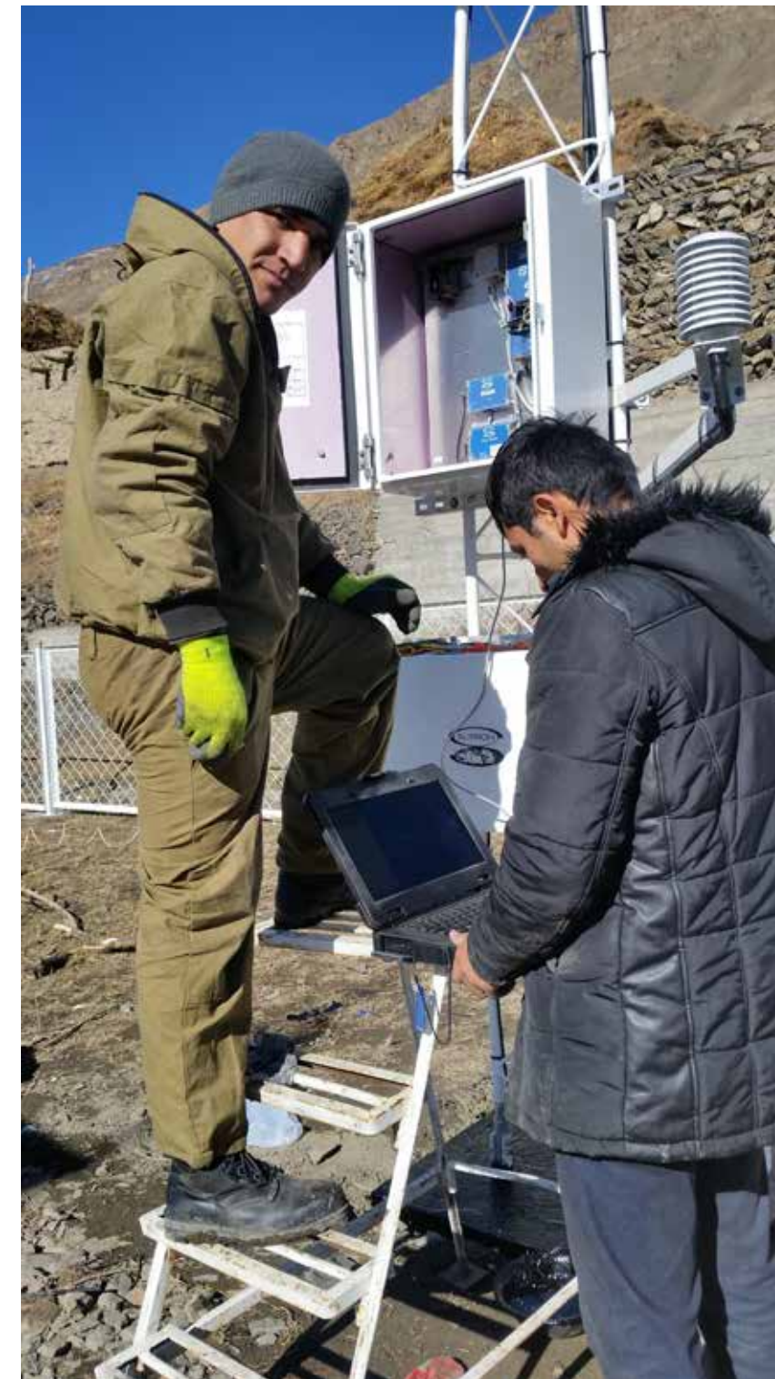
Installation of new equipment, Tajikistan
