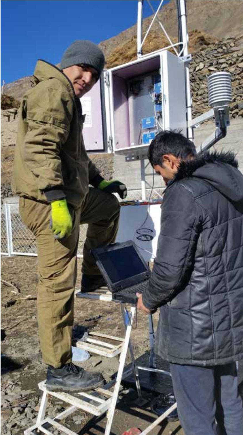
Installation of new equipment, Tajikistan
