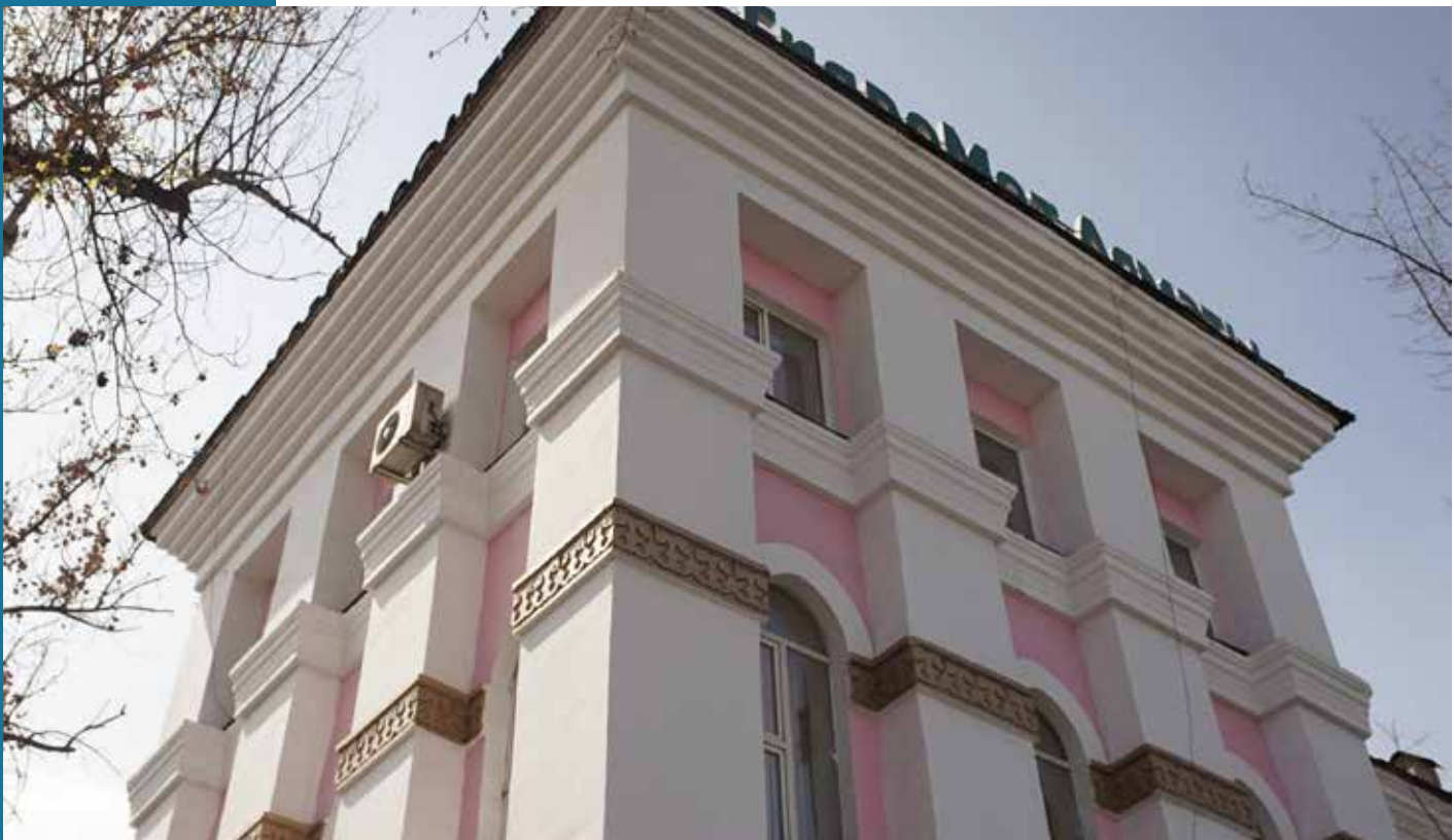
Kaz Hydromet building in Almaty
