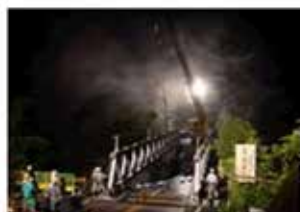
August 4, 2004: Installation of emergency assembly bridge
