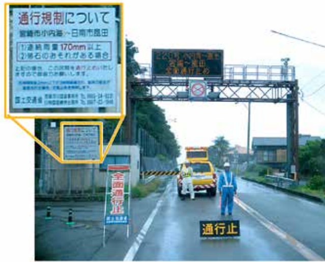
Photo 5.8 Roadside Electrical Information Board with Alarm Light
