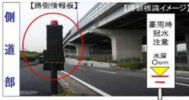
Photo 5.8 Roadside Electrical Information Board with Alarm Light
