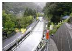
August 5, 2004: Traffic secured on one-way alternating road
