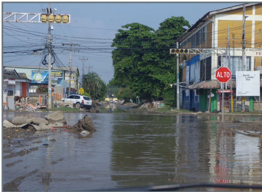
La Lima, Honduras after hurricane Iota. Photo: © Herbert Soriano.
