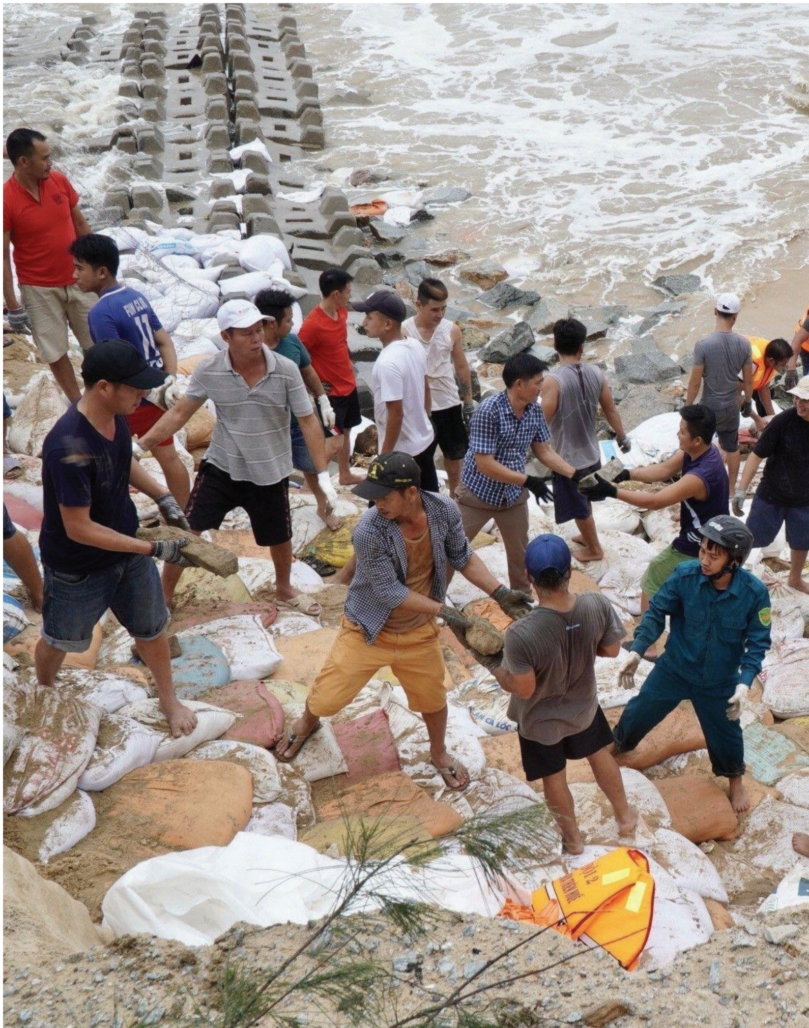
Hanoi, Vietnam. Residents work together to strengthen breakwaters against rising tides caused by heavy downpours Photo: VNA/Xinhua/Alamy Live News.
