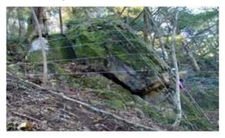
Unstable rock mass is stabilized here using steel wire rope with anchoring to prevent collapse.
