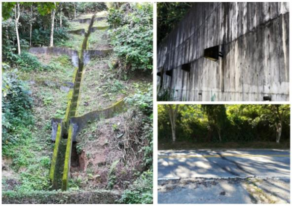
Source: © Javier Escudero Marroquin / World Bank. Further permission required for reuse. Note: "Critical spots" are places that could cause or worsen a potential natural disaster on roads. Clockwise (from left): deteriorated drainage pipe, anchored curtain and bumps on the road due to land movements.
