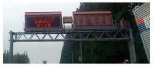
This electronic information board—placed above a carriageway using a bridge structure—announces traffic regulations or conditions. During normal conditions, the electric information board delivers messages that remind vehicle drivers to drive carefully.
