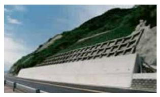
Slope stabilization measures here use a retaining wall, a slope framework (grid beam) with anchoring, shotcrete, and vegetation (bioengineering).
