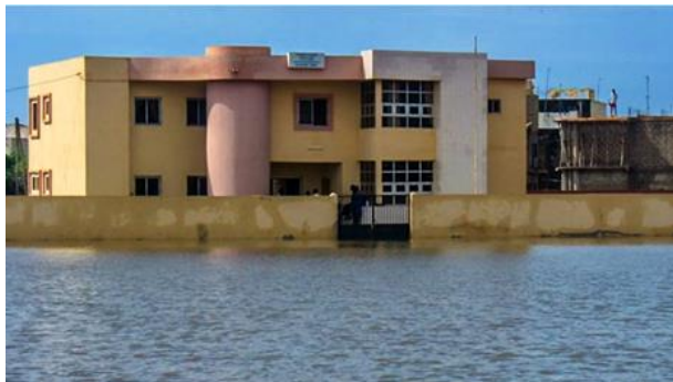
Figure A5.1: Severe flooding in the Dalifort suburb of Dakar (Agence de Développement Municipal).
