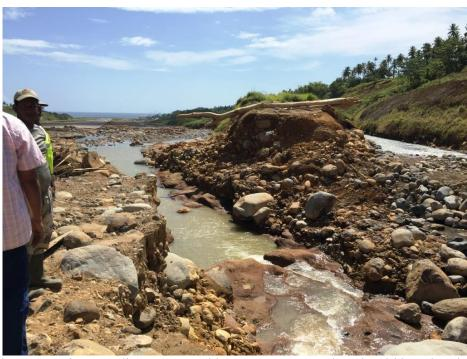
Collapse of Barrage which Caused Inundation of the Airport
