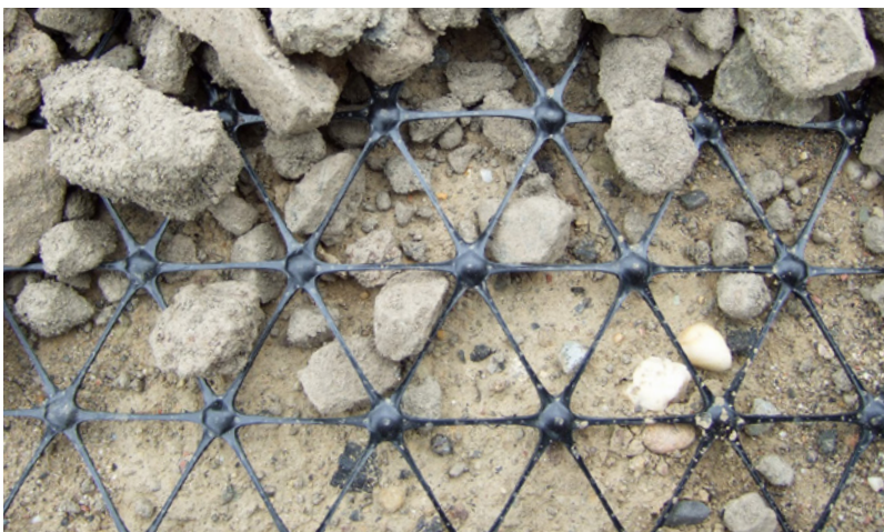
Figure C.14. Typical Geogrid for Use in Bridge Construction
