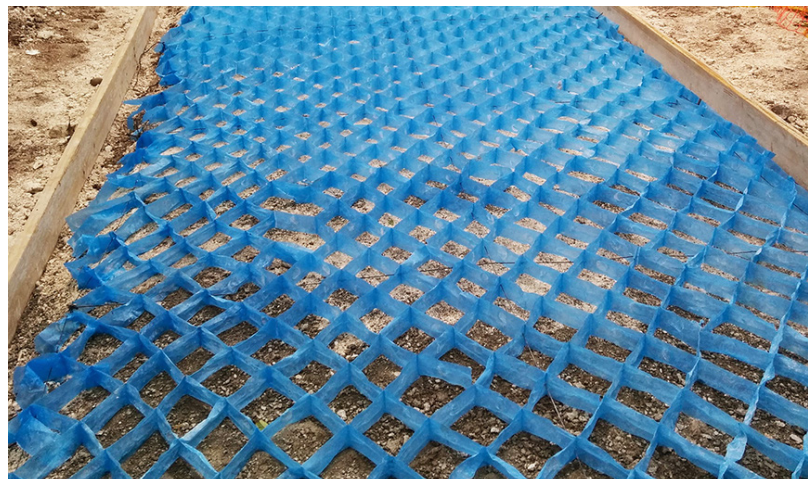
Figure C.8. Geocell Formwork Ready for Placement of Concrete
