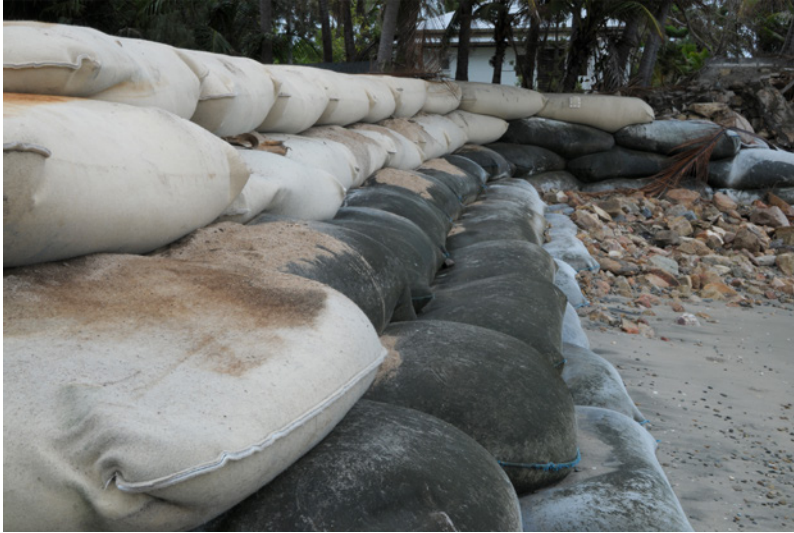
Figure C.11. Geosynthetic Container Revetment
