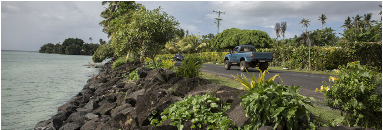
Figure 3.6. Samoa's Vulnerable West Coast Road
