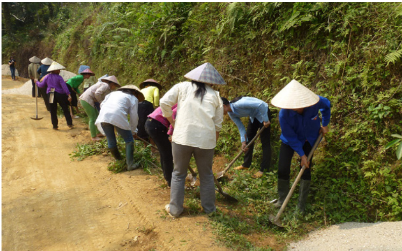
Figure C.26. Construction of a Road Drainage System by Local Communities in Vietnam
