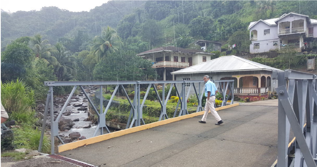
Figure 3.11. Bailey Bridge in Saint Vincent and the Grenadines Purchased under the CERC, 2016
