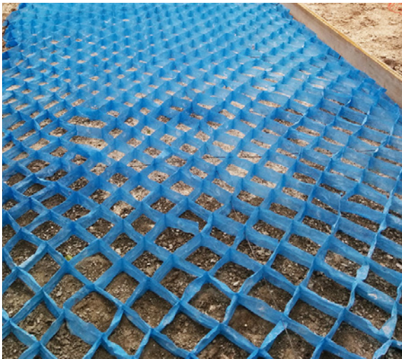
A. Geocell Formwork for Low-Volume Roads in Tuvalu and Kiribati
