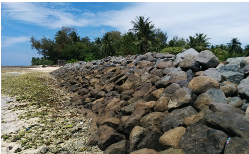
Figure C.10. Rock Revetment in Temaiku, South Tarawa
