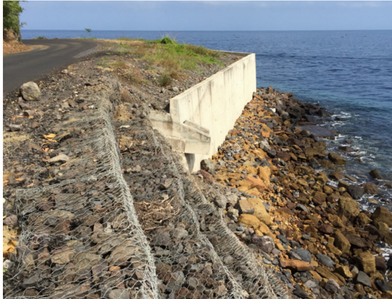
Figure C.29. Slope Stabilization in São Tomé and Príncipe
