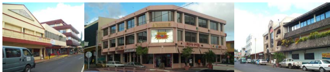
Figure 65: Parts of the Port Vila central business district in the potential inundation zone
