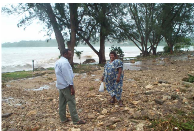
Figure 15: Debris from TC Beni storm waves in harbour-side parking area north of Port Vila CBD
