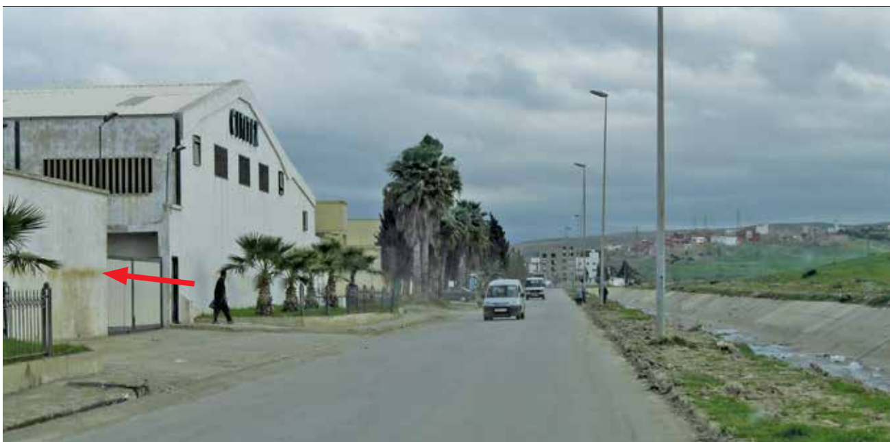
FIGURE 7: Tanger Industrial Zone Flooded in 2008
