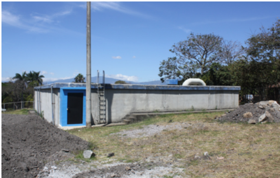
Figure 7 Another side view of the Escazú Cemetery concrete tank. Note the stains left by leaks on the wall.
