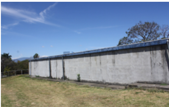
Figure 7 Another side view of the Escazú Cemetery concrete tank. Note the stains left by leaks on the wall.
