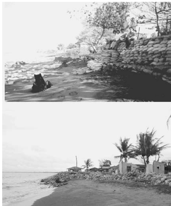
Figure 3. Cheaper alternatives to the more expensive coastal protection structures: sandbags in Wenceslao (top) and ripraps in Alaska (bottom). In the long run, however, maintaining these structures also becomes costly.
