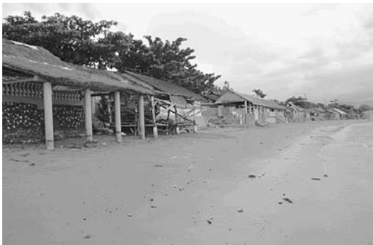
Figure 7. Resorts and restaurants line the southern coast of San Fernando and extends to north of Bauang. These structures provide very narrow shoreline setback for beach adjustment, thereby causing an effect similar to impermeable structures like seawalls and revetments. These photographs were taken in San Vicente; the top photo is the view looking north; bottom is looking south.
