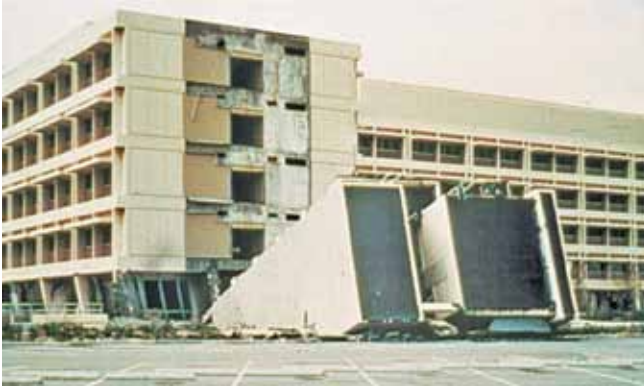
FIGURE 7. The collapsed three month old main building of the Olive View Hospital, San Fernando (Los Angeles, California) M6.7 earthquake of 1971.
