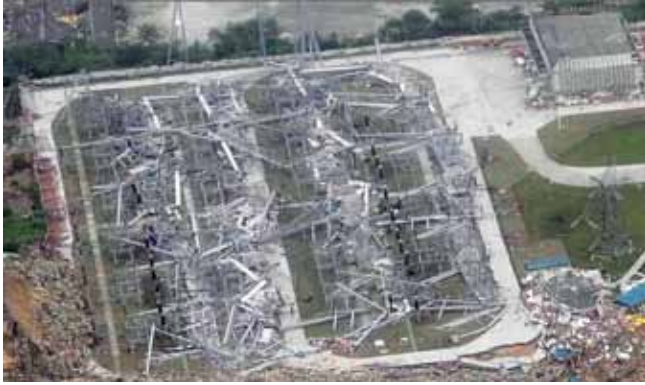
FIGURE 4. Near total destruction of the 220 kV Ertaihan Substation, Yingzhou in the 2009 M7.9 Sichuan, China earthquake.
