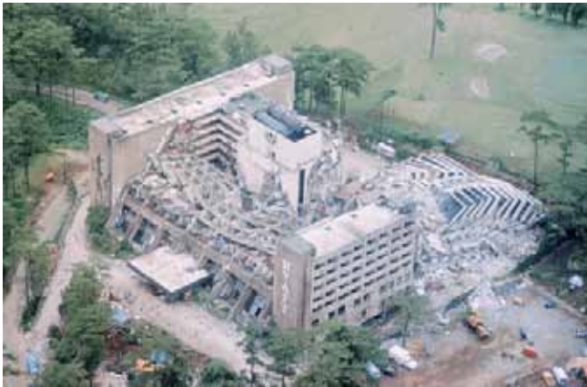
FIGURE 1. One of several collapsed hotels and other modern buildings in the City of Baguio, Philippines; 1990 M7.7 earthquake.
