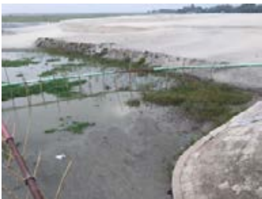
FIGURE 4.7A. ONGOING FILLING OF LOWLANDS IN DHAKA EAST
